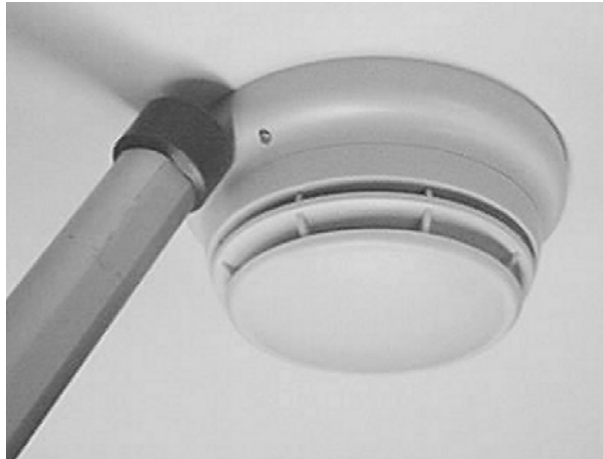
Figure 5-1. Magnet Test Location for 4098-9789, -9791, -9792, -9793, and -9796 Sensor Bases using 553-810 Magnet Tester
