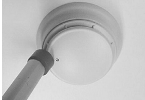
Figure 5-2. Magnet Test Location for 4098-9601, -9602, -9603, -9605 Smoke Detectors using 553-810 Magnet Tester
